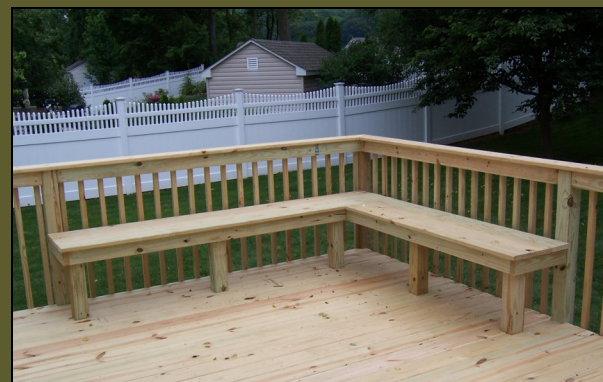
16' x 32' Pressure Treated Deck with Two Sets of Steps and Bench
