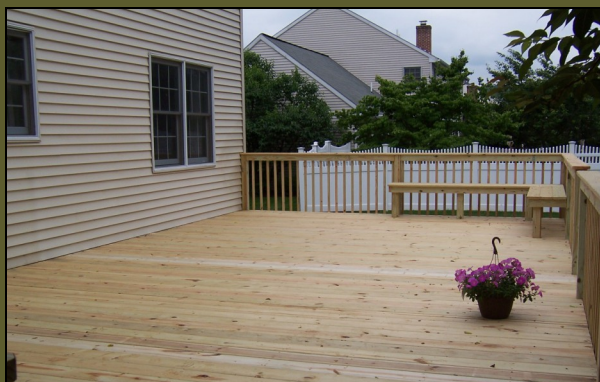
16' x 32' Pressure Treated Deck with Two Sets of Steps and Bench
